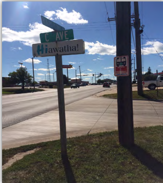
This bus stop at Blairs Ferry and C Ave has developed a beaten path in front from pedestrian travel. Many of the bus stops in the metro area do not have sidewalks connecting to them.
