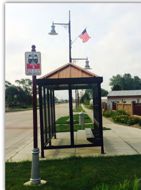
CR Transit bus stop in Hiawatha complete with shelter, bench, bus pad, connection to sidewalk, trash can, and pedestrian lighting.
